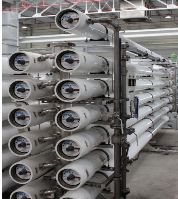
Figure 6. Test vessel mounted atop of a GWRS 5mgd RO unit.
